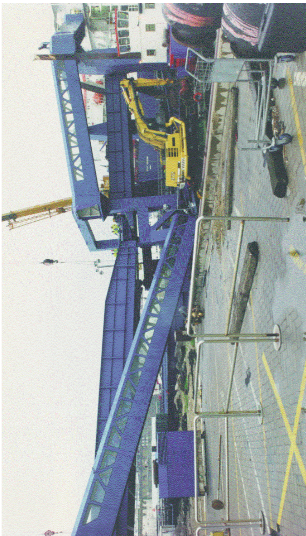
Figure 10: Berth 3 from south west - walkway span in fallen position
