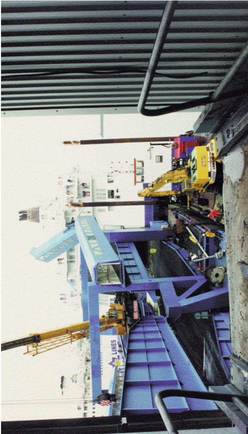
Figure 13: The gap the walkway spanned to the pontoon - and showing ends of passenger ramp slideways
