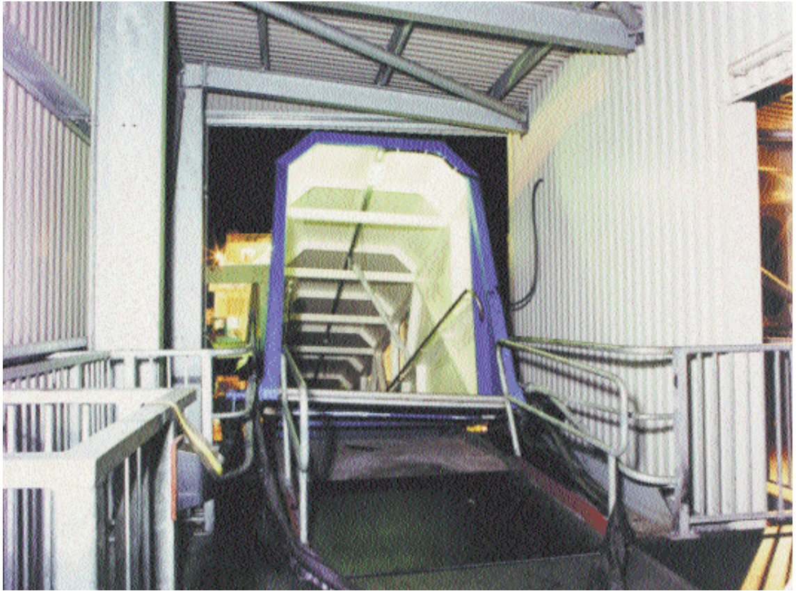
Figure 5: Shore end of collapsed walkway photographed from inside passenger ramp building
