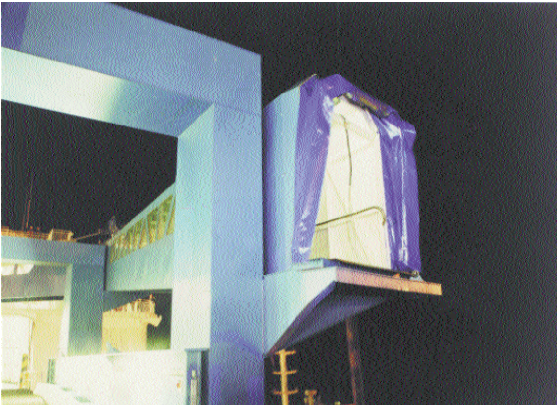
Figure 12: Pontoon support platform and fixed section of walkway
