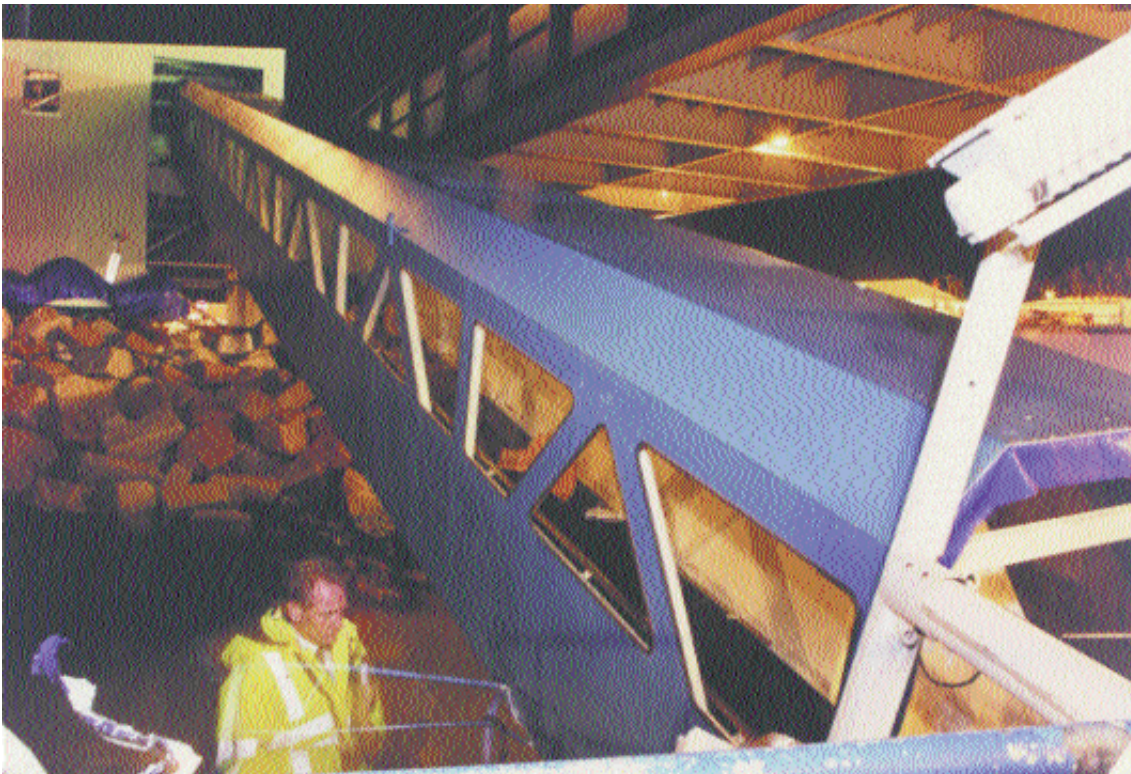
Figure 11: Collapsed walkway from pontoon deck
