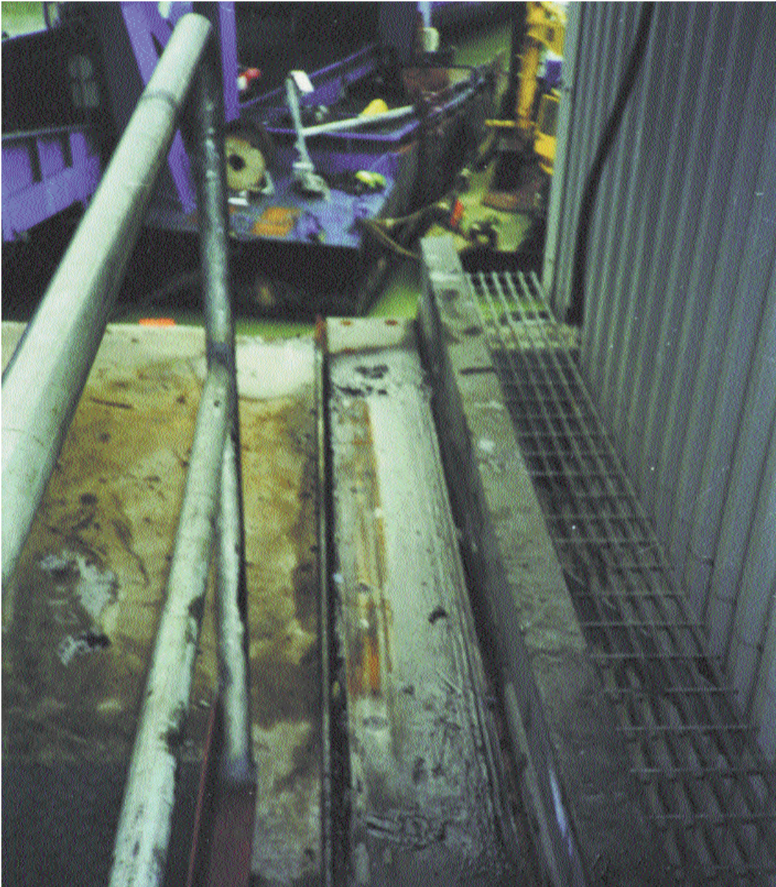
Figure 22: Right-hand slideway in passenger building showing rusting
