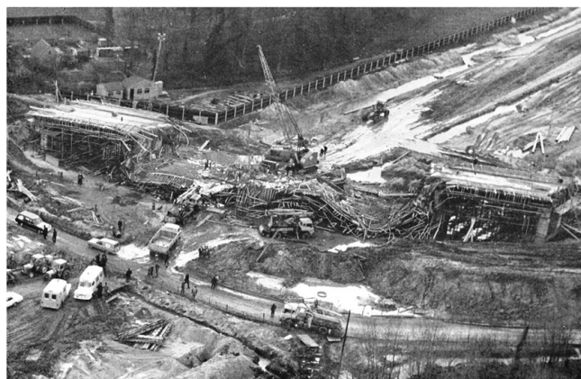
Figure 1. Birling Road, UK, collapse in March 1971 (HSE, 1976)
