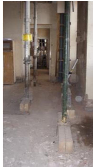
Aluminium props 44Kg each (including jacks)
