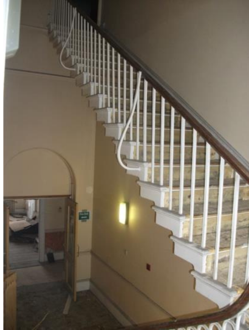
Cantilever stone staircase in the Crescent
