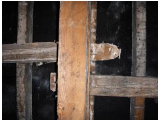
Typical purlin to rafter connection Tusk Tenon + wedge
