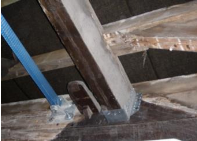
Ratchet strap and hanger at purlin location
