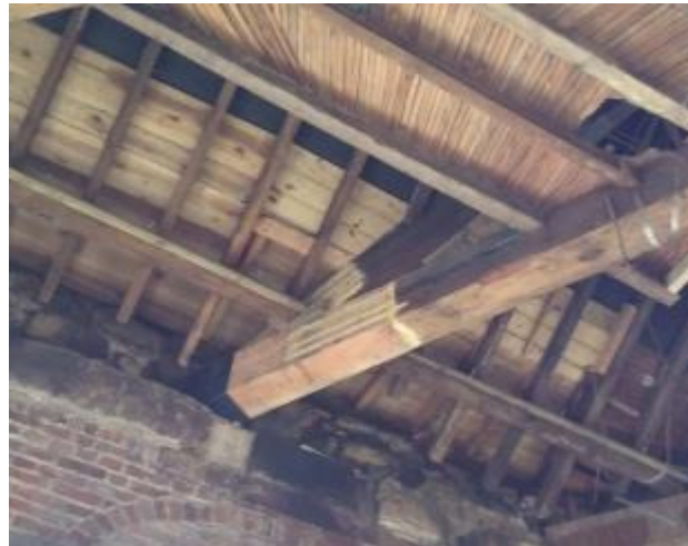
Typical timber resin splice with fibreglass rods
