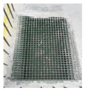
In cases where the permanent works design includes steel riser gratings, if suitable cast-in rebates are designed within the floor slab they can provide support for both the temporary and permanent riser protection. This is preferable to drilled and bolted supports which have to be installed within the riser once the floor slab and core have been cast, before striking the formwork below
