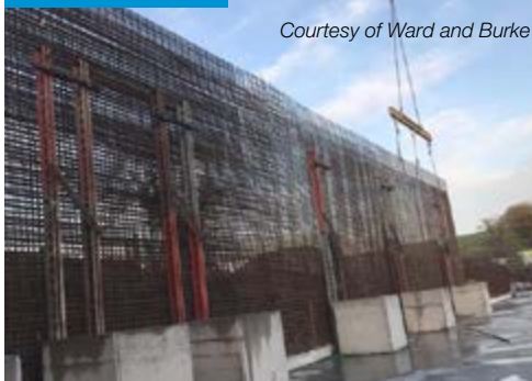
Figure 18: Examples providing stability to cages NOTE: Generally, these details are sacrificial. However, a support frame may be manufactured from proprietary components or from fabricated steelwork and re-used.
