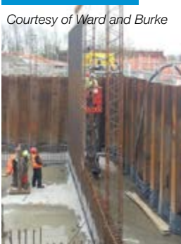
Figure 18: Examples providing stability to cages NOTE: Generally, these details are sacrificial. However, a support frame may be manufactured from proprietary components or from fabricated steelwork and re-used.
