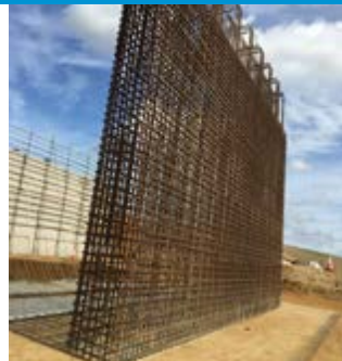
Figure 17: Examples of designed cage supports
