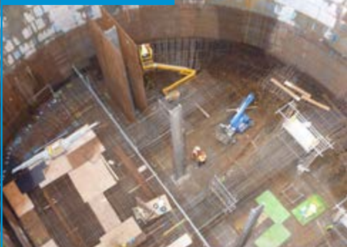
Figure 18: Examples providing stability to cages NOTE: Generally, these details are sacrificial. However, a support frame may be manufactured from proprietary components or from fabricated steelwork and re-used.
